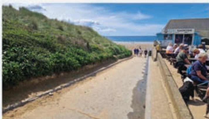
Concrete ramp from car park to the beach. Approx 25m long and sloped.
