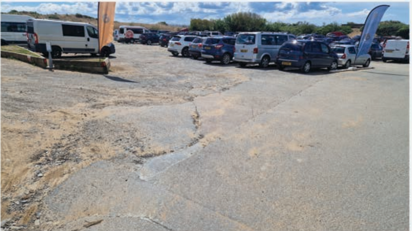
Representation of car park surface - tarmac on the right, hard packed gravel and sand on the left
